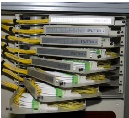
Swing out tray at splitter panel designed for good cable management
