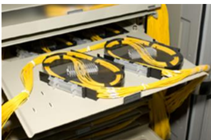
Swing out tray at splitter panel designed for good cable management
